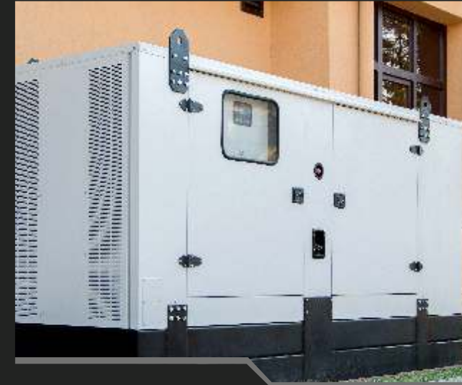
24X7 Power Back-Up
